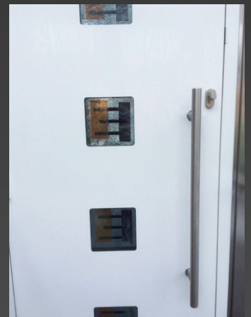
Internal view of door
