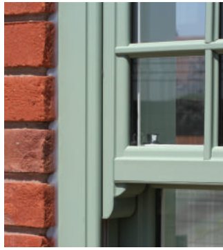
Run through sash horns
